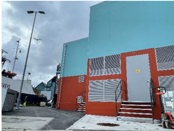
New trafo- and converter building
